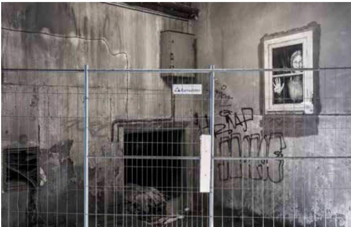
Slussen during demolition. With a graffiti artwork. Photo: Mattias Ek. Stockholm City Museum.
