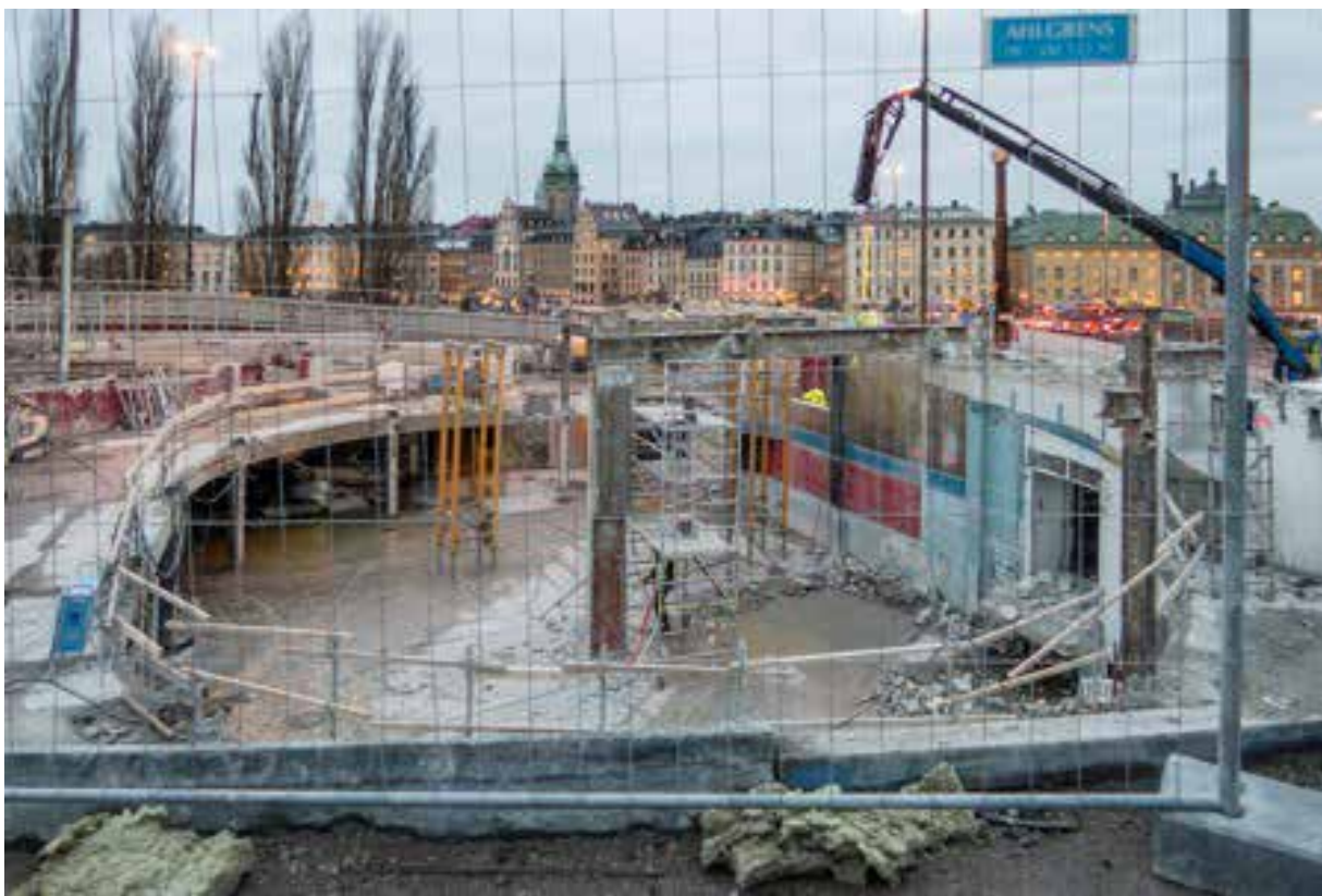
Kolingsborg is torn down. Photo: Matthias Ek, 2015. Stockholm City Museum.
